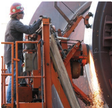
Tire grinding
